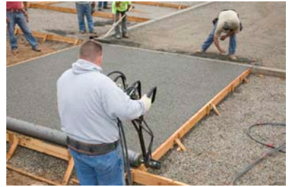
Pervious concrete placement with Roller Screed. November 08
