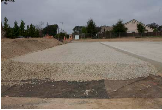
Parking lot stall preparation for pervious concrete including rock placement to ensure a hold area for storm water as it percolates with black geotextial fabric to ensure even settling. November 08
