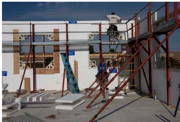
View of inside building during PolySteel production August 08
