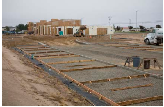
Parking lot stall preparation for pervious concrete including rock placement to ensure a hold area for storm water as it percolates with black geotextial fabric to ensure even settling. November 08
