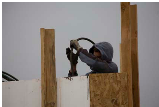
Pencil vibrator used to consolidate concrete in PolySteel wall September 08
