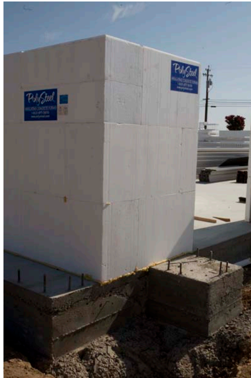
Corner view of PolySteel wall August 08
