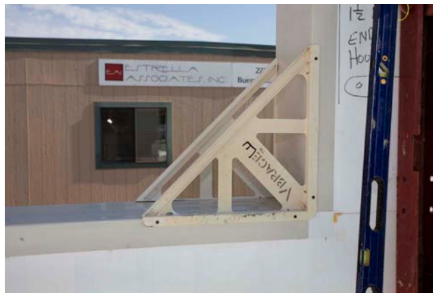
Window opening in PolySteel wall preparing for concrete pour August 08
