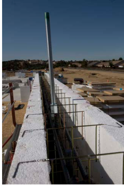
Westside wall stacked with PolySteel - River Oaks Center August 08
