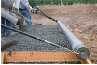
Pervious concrete placement with Roller Screed. November 08
