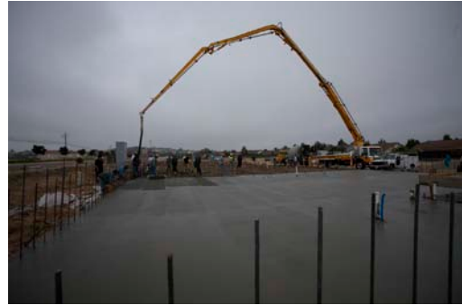
Concrete boom-pump providing concrete for the main building slab July 08
