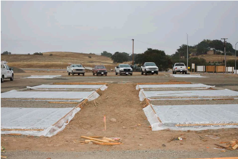
Pervious concrete parking stalls covered and ready to cure. November 08
