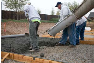
Pervious concrete placement with Roller Screed. November 08
