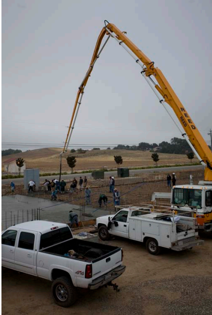
Bird's eye view of concrete placement July 08
