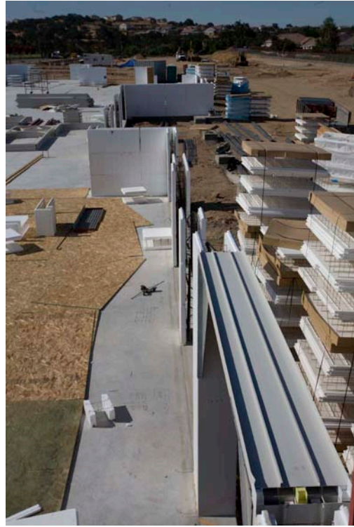
Elevated image of River Oaks Center with PolySteel walls August 08
