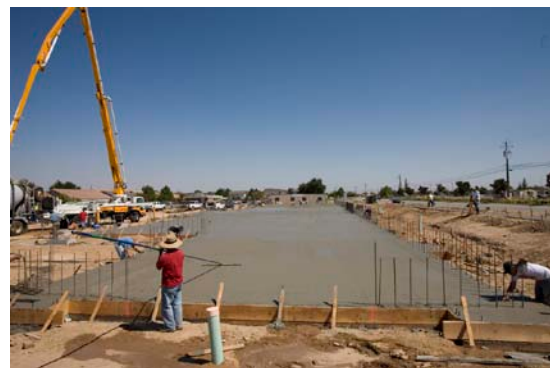
Completing southern portion of building slab July 08
