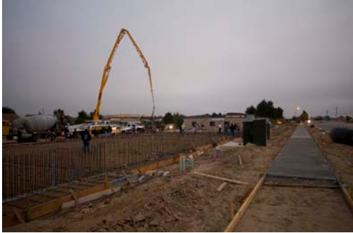
Placement of concrete for main building slab July 08
